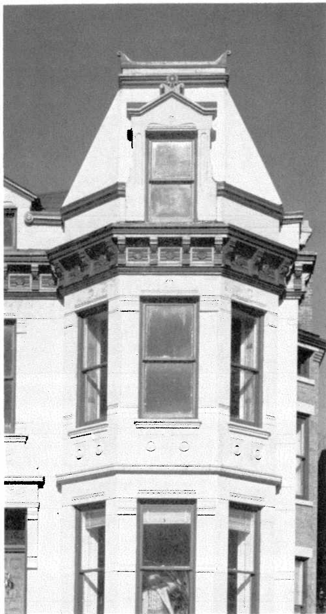
Bay-front building at 1520 West Jackson is enriched with the ornament of the Second Empire style. Note the mansard roof with the prominent dormer window.
